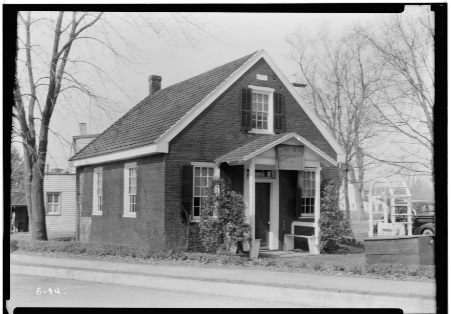
1936 photo of the Clara Barton Schoolhouse showing that the bricks and mortar were painted (red).
